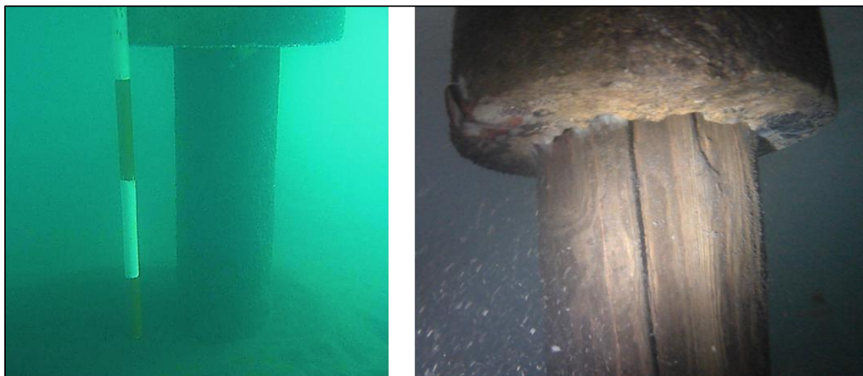
Figure 2.3 A wooden pile submerged in Hévíz lake (Author).
